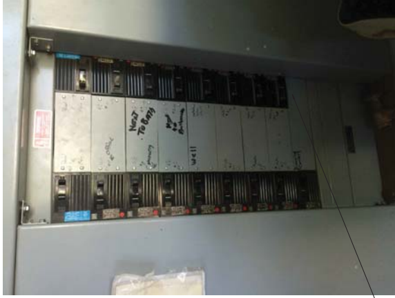
EXISTING SPACE FOR NEW CLASSROOM BUILDING CIRCUIT BREAKER.
